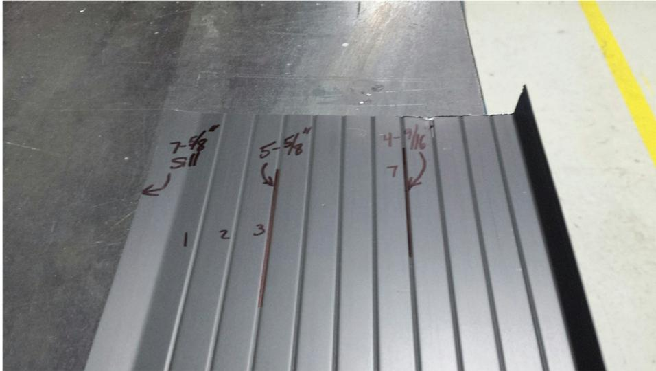
***TIP:** The sill cover has been designed to work with Quanex (Imperial) sills. For your convenience, we have designed the treads act as cutting guides for your knife.*
